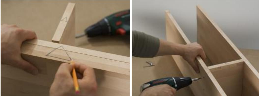
Arrange the two upper shelf panels and the centre side panel on their leading edges to form a double T-beam in the way you want to screw them together. Now use a pencil to mark the rear edges so that you always know what goes where at a later stage of assembly. Carpenters normally use a triangular symbol for this purpose.
