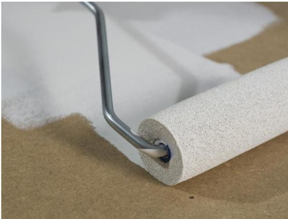
To achieve a perfect finish on your furniture, paint the sections before assembly. First read the manufacturer's safety and handling instructions thoroughly. Make sure the room you are working in is well ventilated and not used for smoking, eating or drinking. Apply the priming filler with the roller or with a paint spraying system if necessary. Allow it to dry completely.
